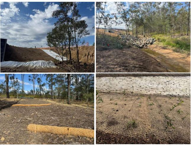
Photo set 4: Erosion, sediment and drainage controls installed within open space and retained vegetation areas.
